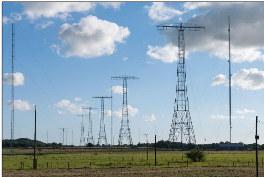
LF Antenna at World Heritage Grimeton Radio Station
