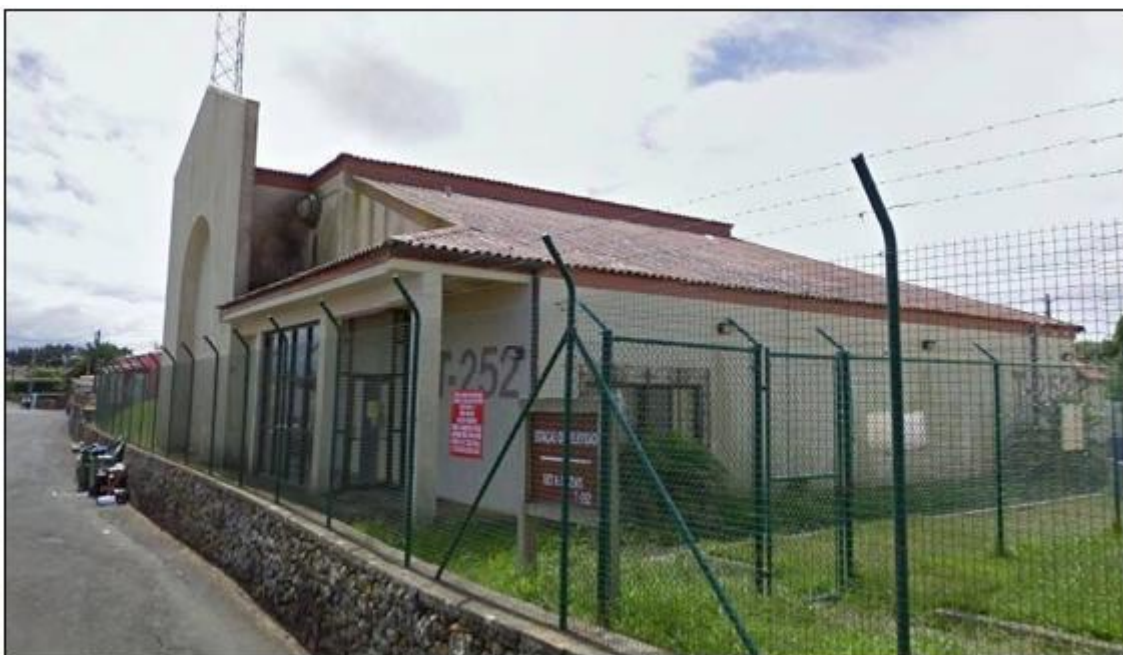
The AFRS CSB 83 building. (Picture: AFRTS)
