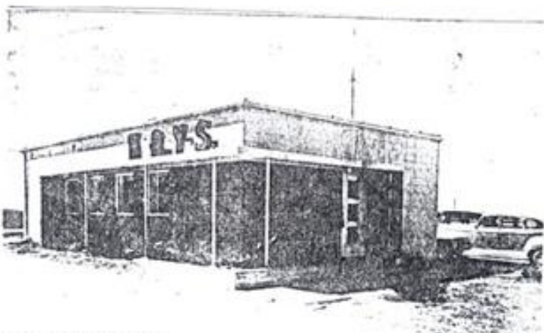
LOOKING NORTH WEST
